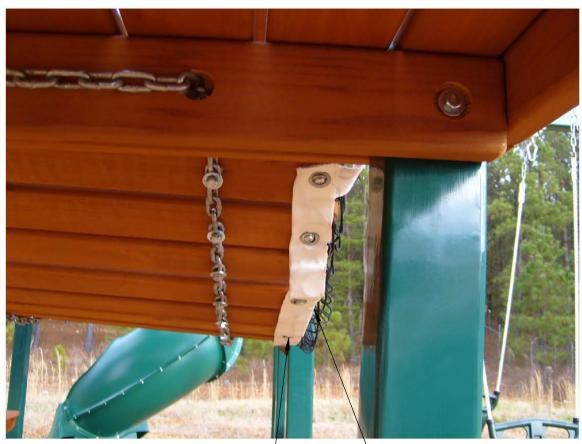
MARK THROUGH THE CENTER OF THE CENTER GROMMET ONTO THE MIDDLE DECK BOARD. DRILL A 1/8" X 1" DEEP HOLE AT THE MARK. PLACE A PAN HEAD SCREW THROUGH A WASHER AND INSTALL INTO THE HOLE. TRY TO CENTER THE WASHER ONTO THE GROMMET BEFORE TIGHTENING COMPLETELY.
